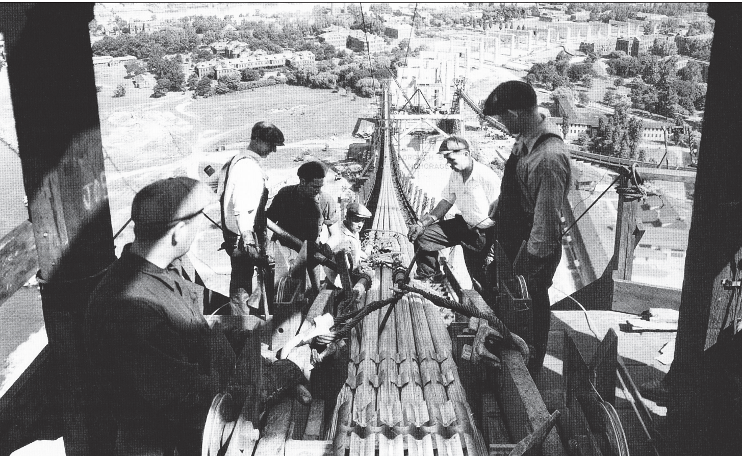
Workers laying cable on the Triborough Bridge – built as a New Deal project. NYLHA's Spring Labor History Conference, When Government Was the Solution: The New Deal's Forgotten Legacy – June 8. (Boxed entry below.) 1935 photo courtesy of The New York Public Library Picture Collection.
